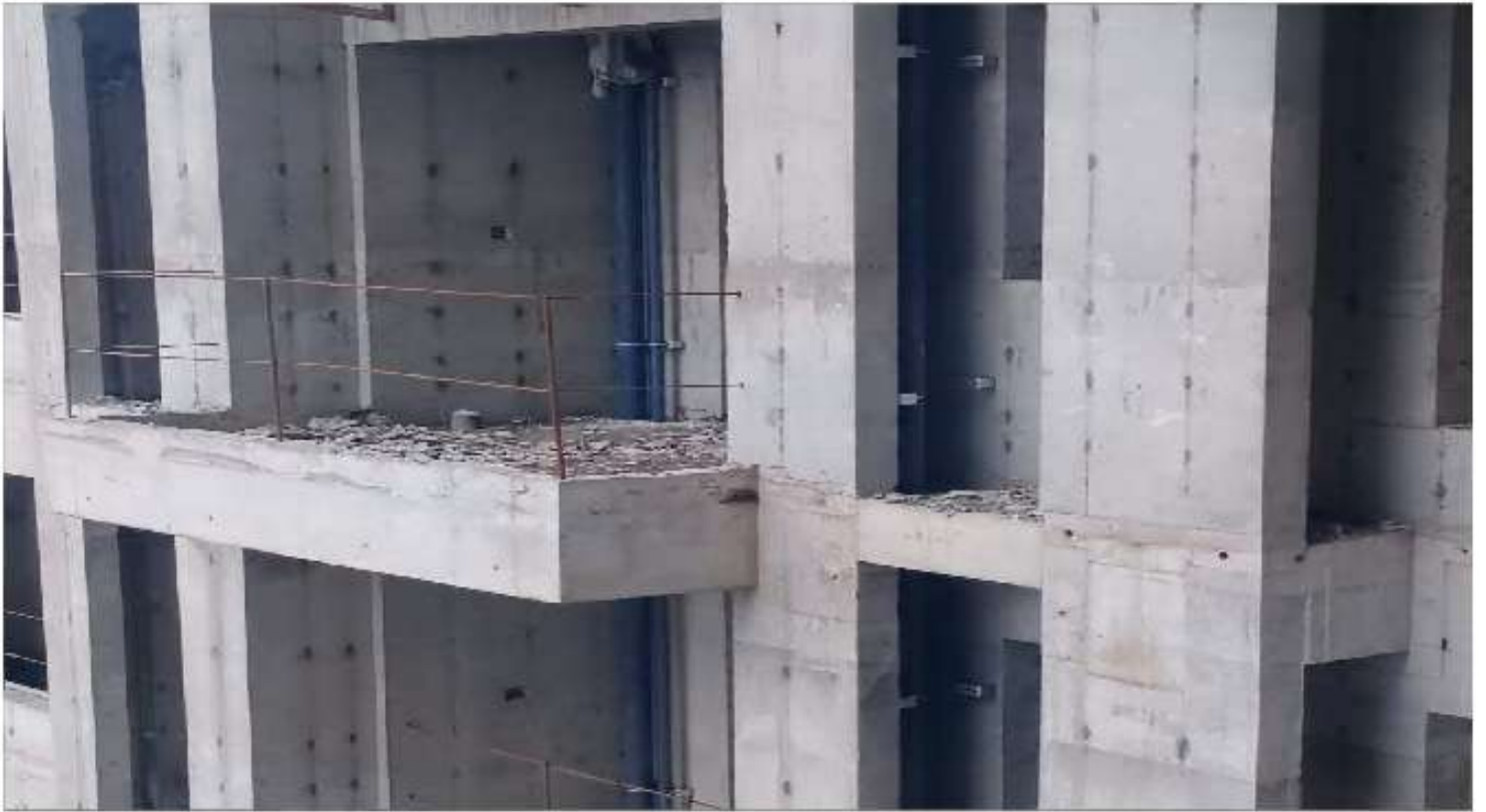
TOWER-2, OUTER DUCT AND INTERNAL PHE WORK IN PROGRESS
